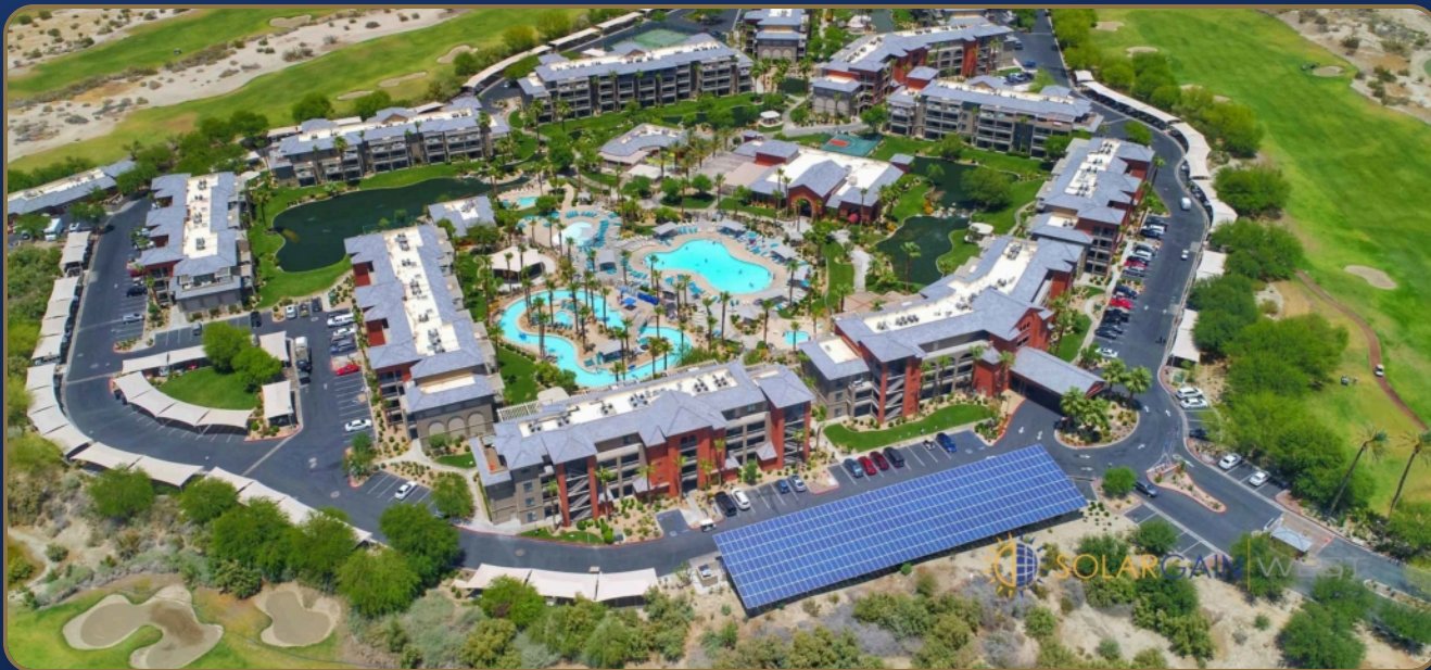
CARPORT SOLAR ARRAY • SOLAR GAIN COMMERCIAL INSTALLATION
